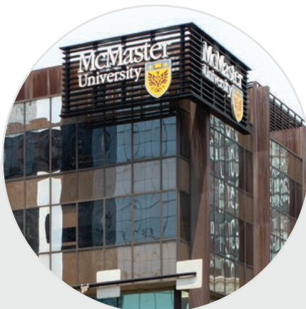
McMaster's One James North Building
